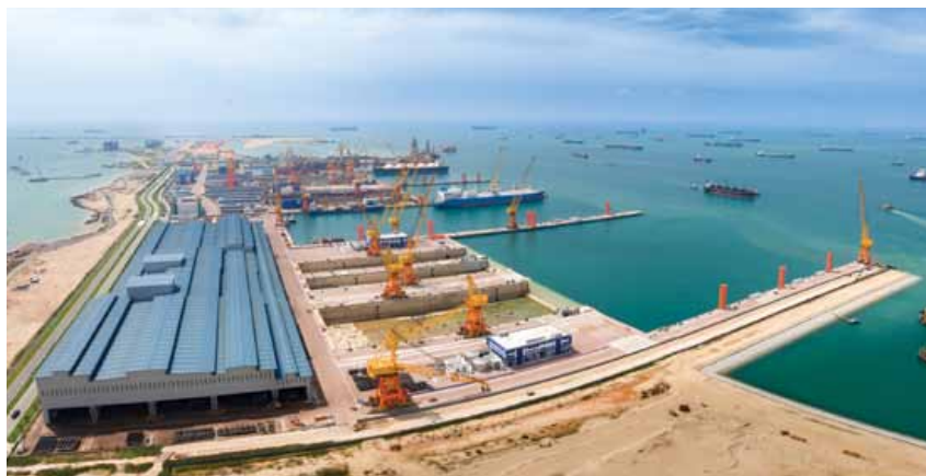
Sembcorp Marine Tuas Boulevard Yard Phase II development was completed in January 2017
