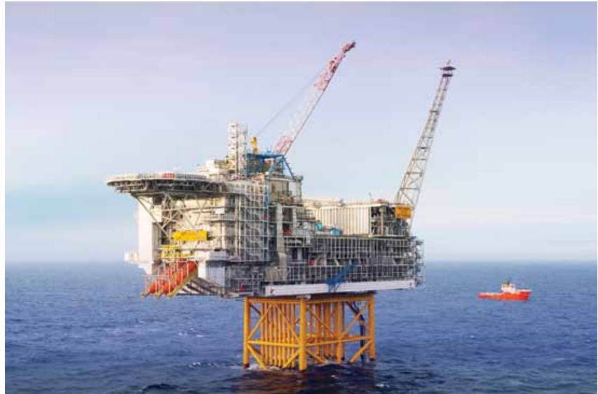
Sembcorp Marine delivered the Process, Drilling and Quarters (PDQ) platform topsides to Det norske oljeselskap ASA (now part of Aker BP ASA) for the Ivar Aasen field development in the North Sea
