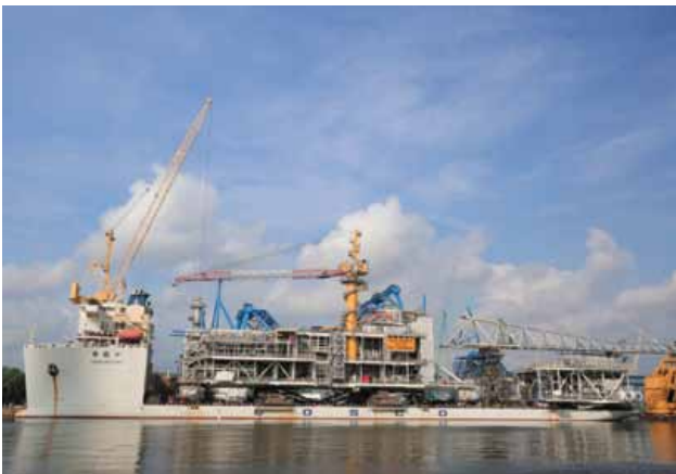
Completion of Ivar Aasen process, drilling and quarters platform project
