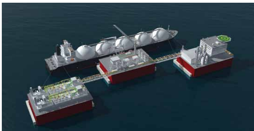
A Gravifloat LNG liquefaction plant and export terminal, with capacity to handle 2 to 3 million tonnes of LNG per year
