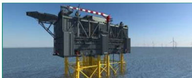
Sofia Offshore Wind Farm Project: Design, construction, installation and commissioning of Offshore Converter Platform for RWE Renewables
