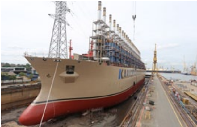
Power ship refits underway
