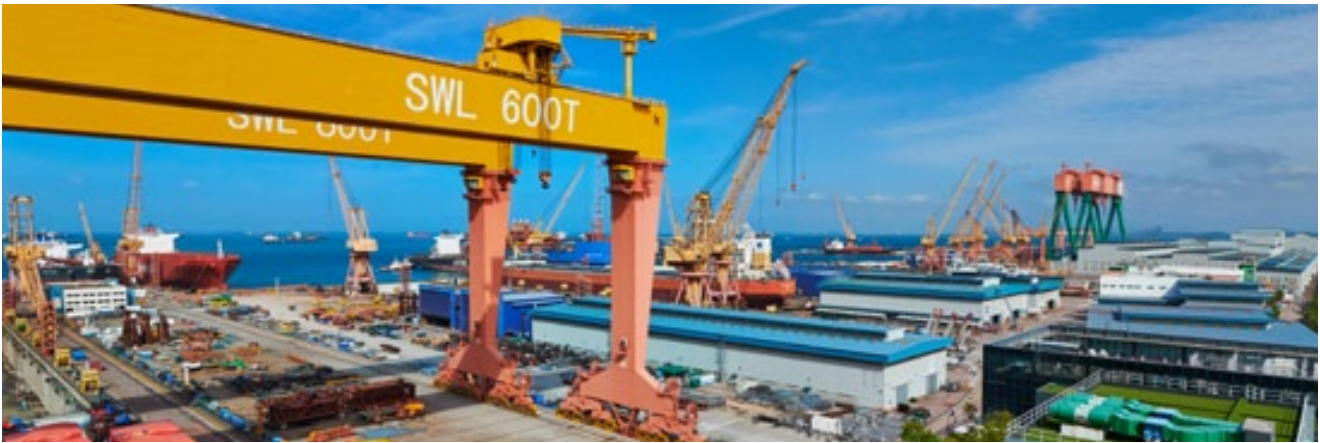
Various marine and offshore projects underway at Tuas Boulevard Yard
