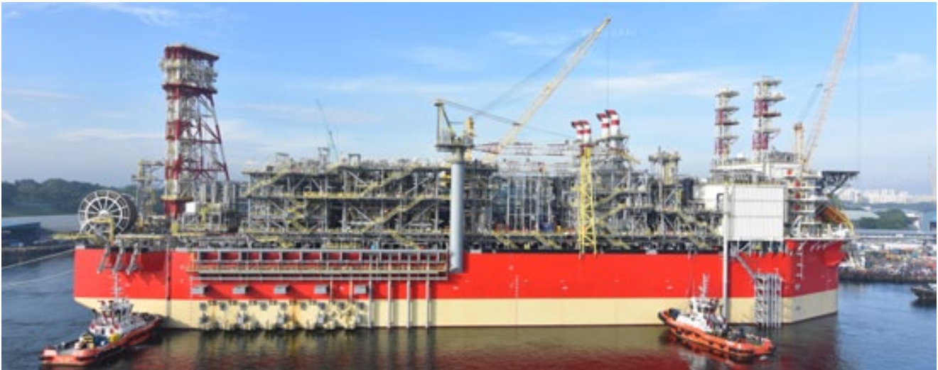
Sailaway of newbuild FPSO Energean Power following successful construction for operation in the Karish Field in the Eastern Mediterranean
