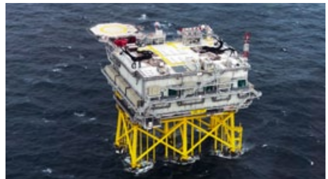
The Group has secured the Planned Preventative Maintenance contract to maintain and service the low voltage and ancillary systems for the Hornsea 2 Offshore Wind Farm OSS and RCS platforms following the project's successful delivery
