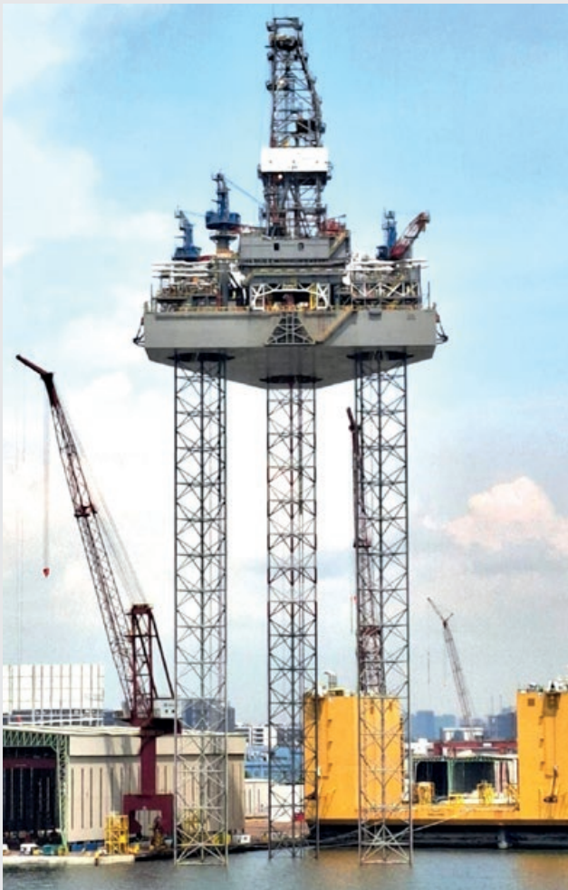
Var - the final unit in a series of five B Class jack-ups delivered to Borr Drilling
