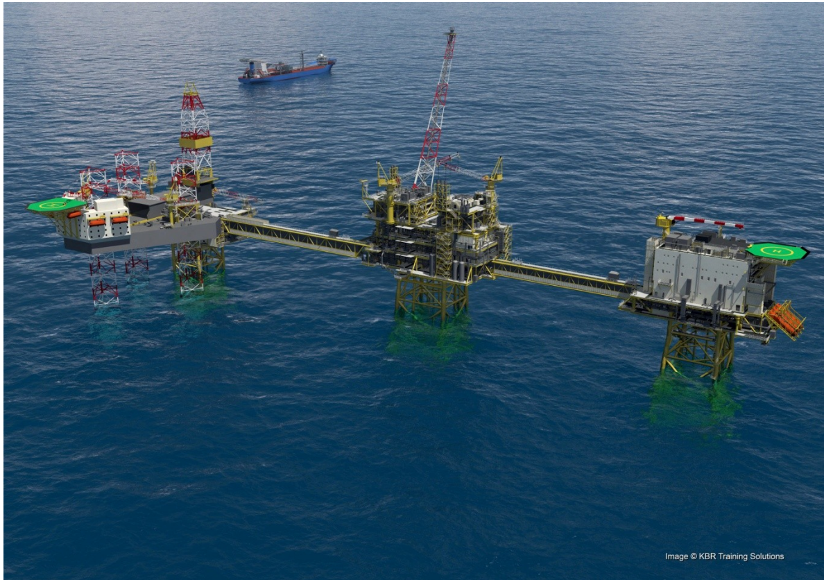
Caption: The contract includes the building of the Central Processing Facility plus 2 connecting bridges, Wellhead Platform and Utilities & Living Quarters Platform Topsides for the Culzean Field Development. The facility will be installed at a water depth of some 90 meters in the UK sector of the Central North Sea.
