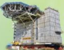
EPC of North Sea-ready living quarters, flare and bridge
