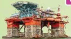
Repair and upgrading of an accommodation semi-submersible rig
