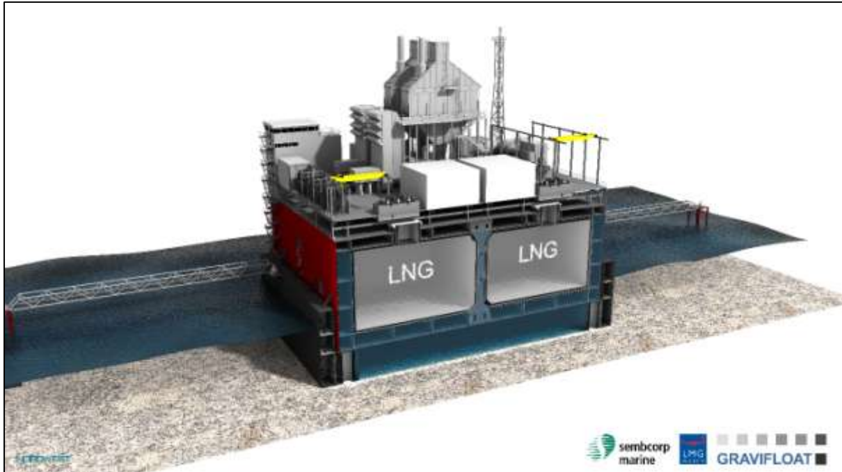
Caption: Sembcorp Marine and ENGIE will develop a Gravifloat 3-in-1 integrated solution for near-shore receiving, storage and regasification of LNG as well as power generation.
