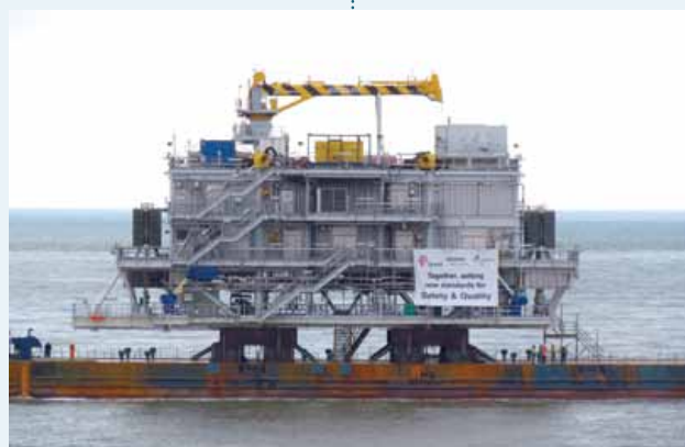
Dudgeon Offshore Wind Farm Substation Platform
