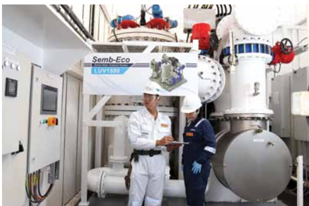
The environmentally-friendly, energy-efficient Semb-Eco LUV is the first IMO type-approved ballast water treatment system in Singapore
