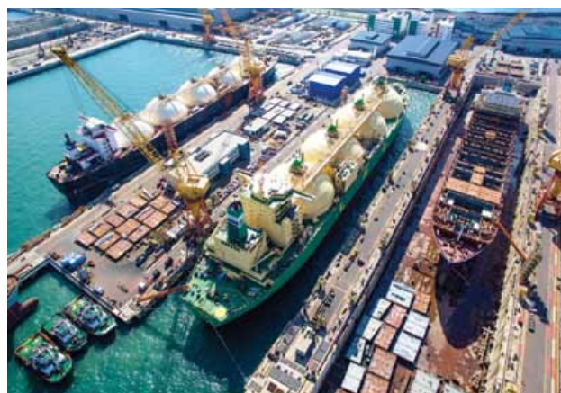
Containership and LNG carriers undergoing repair and overhaul work at the Sembcorp Marine Tuas Boulevard Yard
