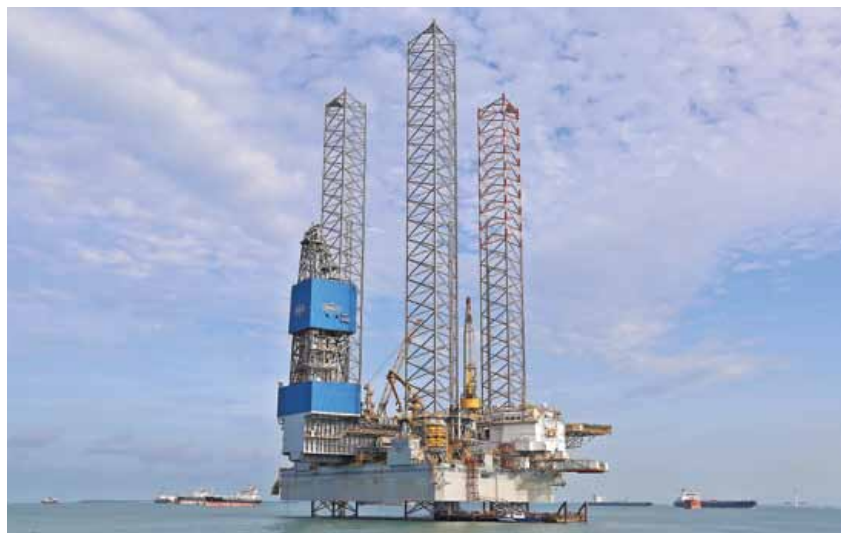
For deployment at Statoil's Mariner field development in the North Sea, Noble Lloyd Noble is the first offshore structure of its kind to fully comply with both Norwegian and UK regulatory standards
