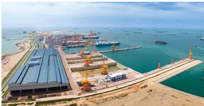
Sembcorp Marine Tuas Boulevard Yard Phase II development was completed in January 2017
