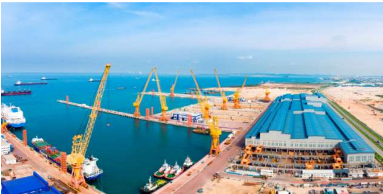
Southeast Asia's largest single solar rooftop at a shipyard will be installed atop Sembcorp Marine Tuas Boulevard Yard's steel structure fabrication workshop (building on the right with blue roof)
