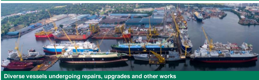
Diverse vessels undergoing repairs, upgrades and other works
