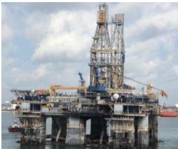
Repair of semi-submersible Noble Clyde Boudreaux
