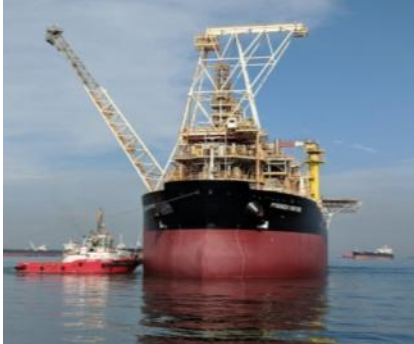
Major upgrading of FPSO Pyrenees Venture for MODEC / BHP Billiton
