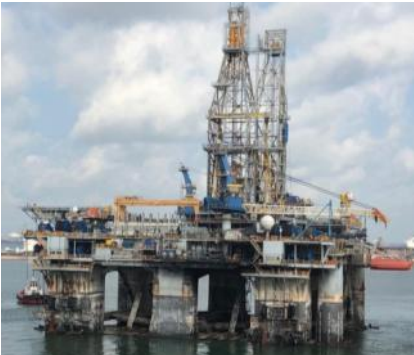
Repair of semi-submersible Noble Clyde Boudreaux
