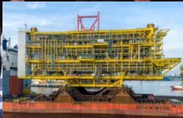
Well Head Fixed Platform Topside (Admiralty Yard, Singapore)
