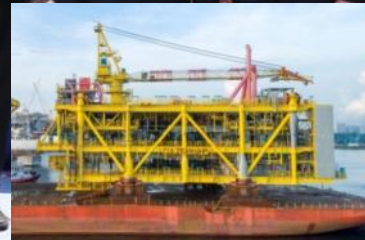
Central Processing Facility Fixed Platform Topside (Admiralty Yard, Singapore)
