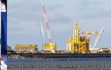
Power Generation Module & 2 Interconnecting Bridges (Sembmarine SLP, UK)
