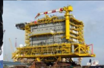
Utilities & Living Quarters Fixed Platform Topside (Admiralty Yard, Singapore)
