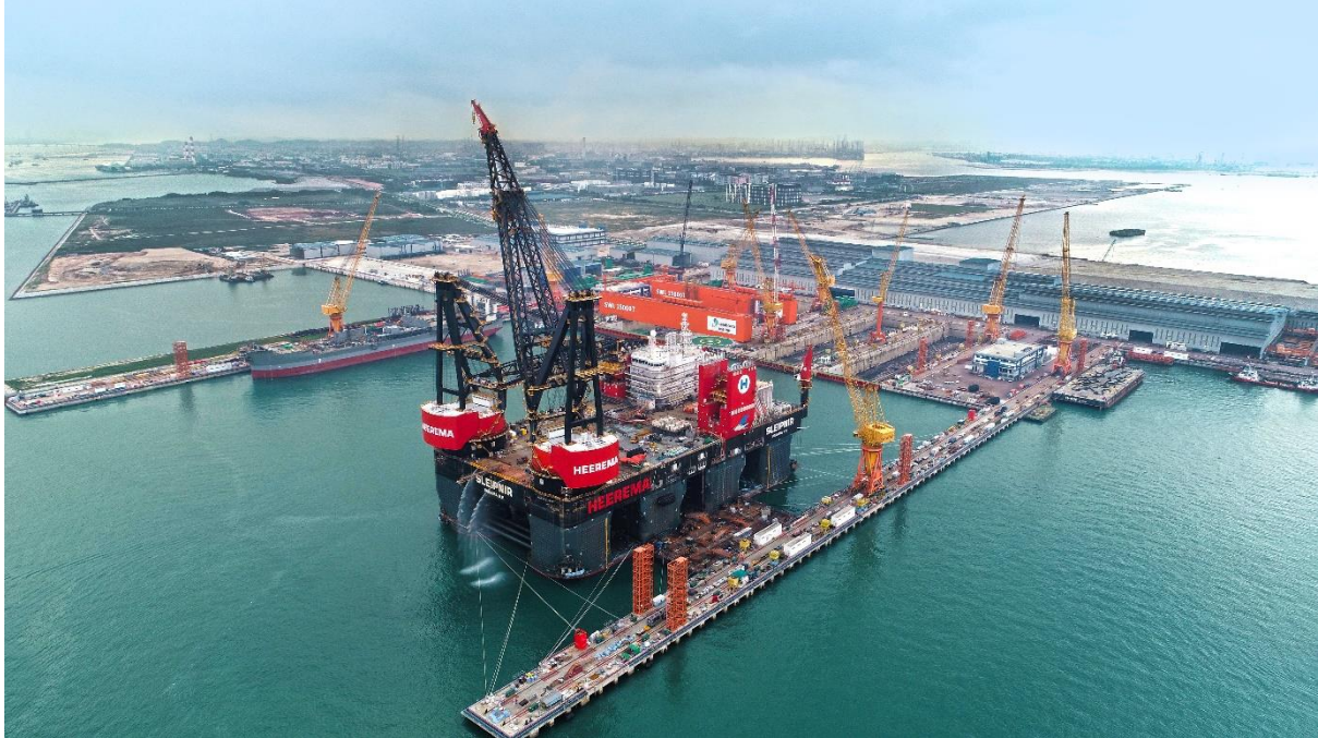
Sleipnir, the world's largest and strongest semi-submersible crane vessel built by Sembcorp Marine (a)
