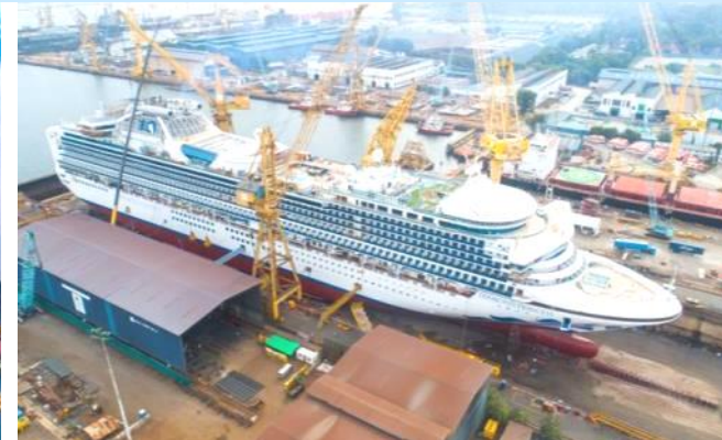
Repairs and installation of scrubbers on Diamond Princess for Princess Cruises
