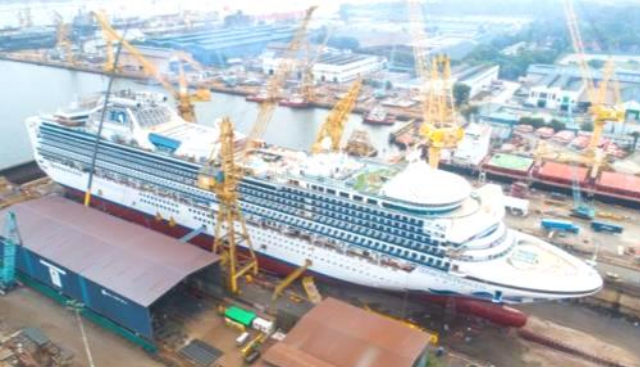
Repairs and installation of scrubbers on Diamond Princess for Princess Cruises
