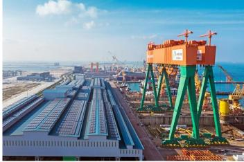
Solar panels (left) at Sembcorp Marine Tuas Boulevard Yard powers the Group's steel fabrication facility with clean energy. On the right is the Yard's goliath cranes with 30,000 tonne lifting capacity and 100m hook height that enable mega-block installation, helping customers fulfil business objectives of safety, quality, time and cost.
