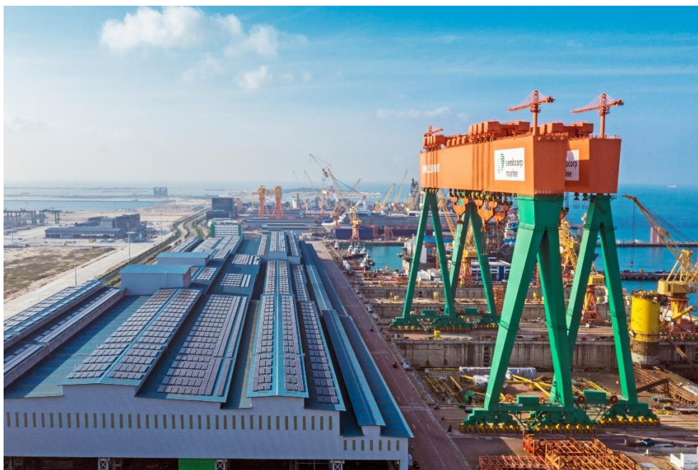
Solar panels (left) on the roof of our steel fabrication workshop at Tuas Boulevard Yard provide clean energy for up to 30% of maximum production capacity. With a capacity of 4.5 MWp, the panels can generate up to 5,000 MWh of clean energy, enough to power some 1,100 four-room flats annually.
