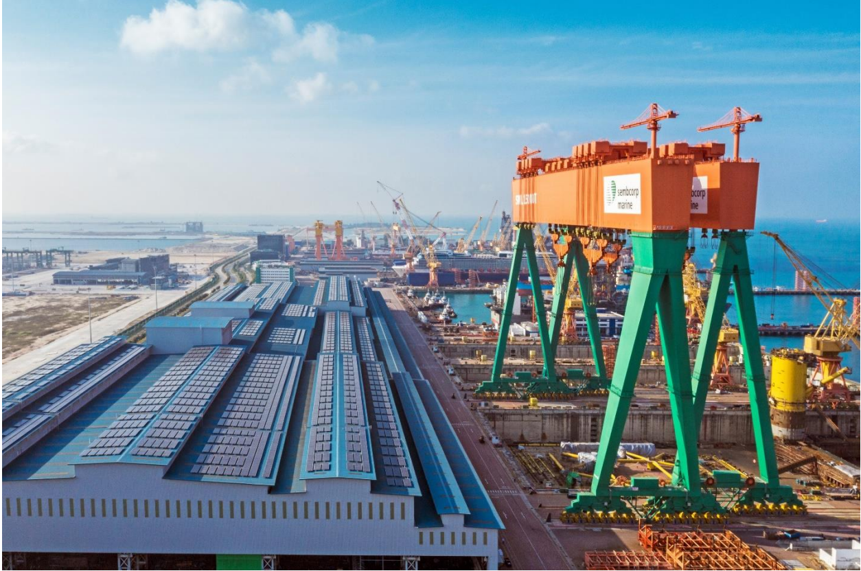
Solar panels (L) installed at Sembcorp Marine Tuas Boulevard Yard during Phase 1 of Sembcorp Marine and SP Power's collaboration
