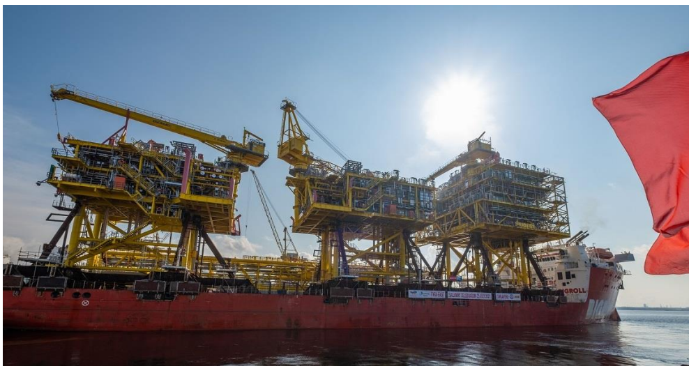
Topsides and bridges of Tyra Redevelopment Project ready for sailaway from Sembcorp Marine Admiralty Yard
