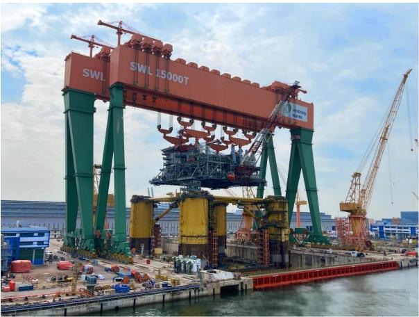
Tandem lift of the Vito Host mega-topside structure onto the FPU hull by a pair of goliath cranes, with combined 30,000-tonne lifting capacity and 100-metre hook height, at Sembcorp Marine Tuas Boulevard Yard.
