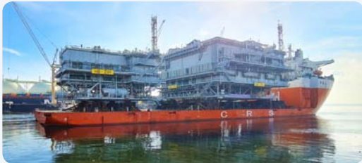
Hornsea 2 Offshore Wind Farm substations
