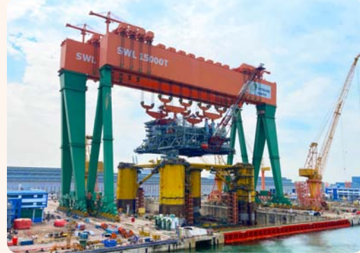
Tandem lift of the Vito RPF mega-topside structure for integration with the FPU hull by a pair of cranes, with combined 30,000-tonne lifting capacity and 100m hook height, at Sembcorp Marine Tuas Boulevard Yard
