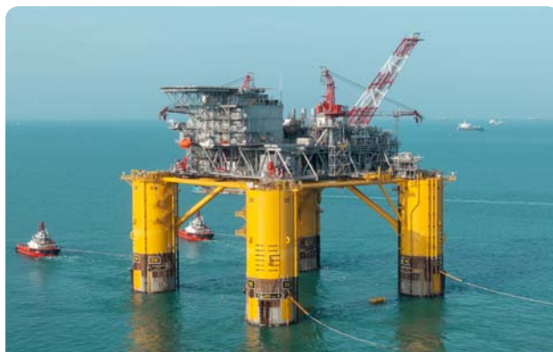
Successful delivery of the Vito RPF – the first of two newbuild FPUs – in December 2021
