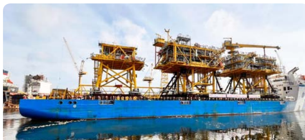
Tyra West modules and bridges delivery
