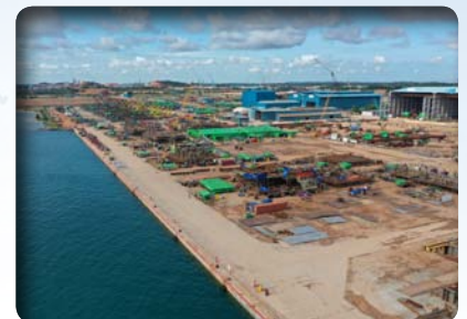
SEBMCORP MARINE BATAM YARD (PT. SMOE INDONESIA)
