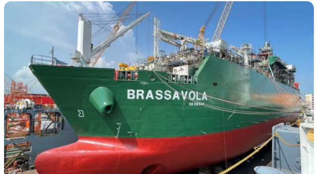
Work is in progress for the newbuild 12,000m³ LNG bunker vessel
