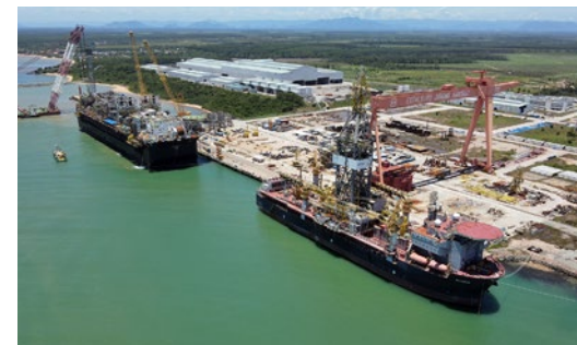
Process Solutions | REPAIRS & UPGRADES Work
