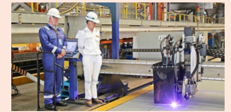
Strike steel to mark construction commencement
