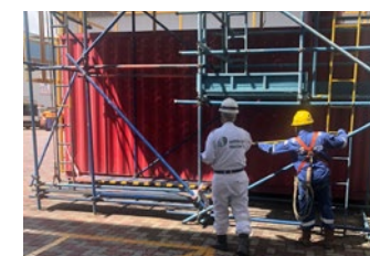
Performing erection and dismantling of cargo hold (tower) scaffold
