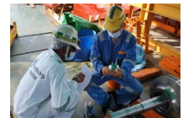
Performing maintenance for pump room
