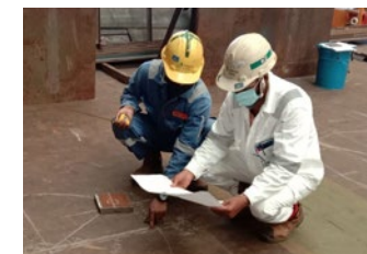
Performing basic outfitting activities measurements
