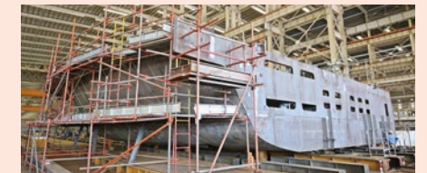
Construction in progress in the highly automated steel fabrication facility
