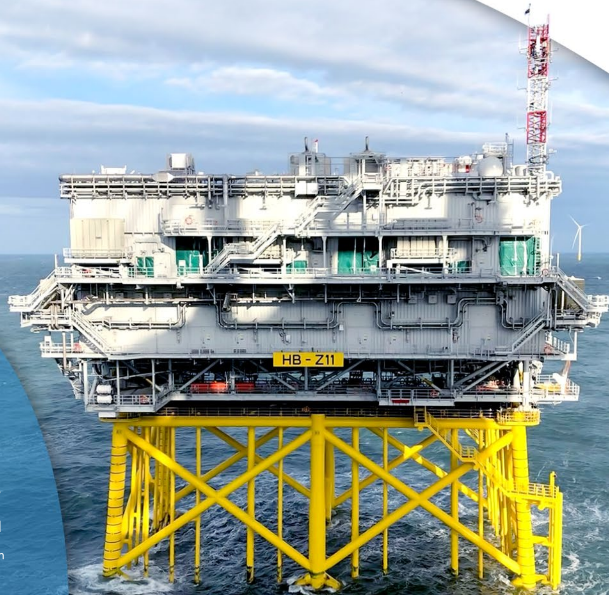
Offshore Substation at Hornsea 2 Offshore Wind Farm
