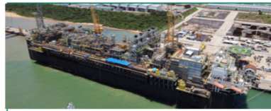
Amendment contract for P-71 by Tupi B.V. to perform modification work and additional topside modules integration for deployment to Itapu Field
