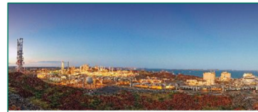
Pluto Train 2 Project: Modules assembly of LNG gas processing trains for Bechtel Overseas Corporation
