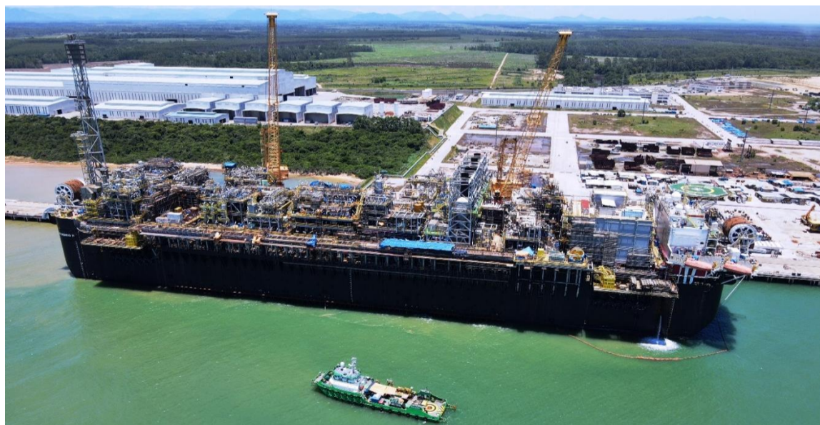
Estaleiro Jurong Aracruz completes P-71, its second FPSO modules fabrication and integration project for Tupi B.V. (Photo: Sembcorp Marine Ltd, all Rights reserved)
