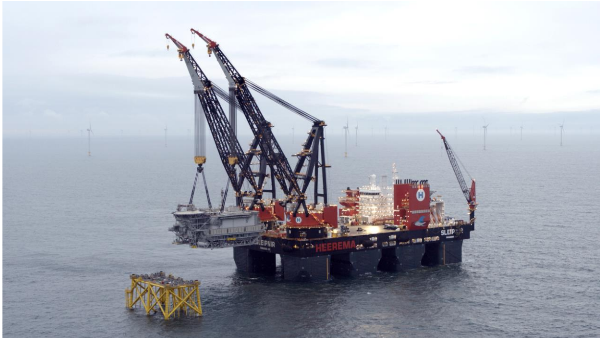
Sembmarine SLP performed the offshore installation, hook-up and commissioning of the Hornsea 2 Offshore Wind Farm platforms, which were fabricated by Sembcorp Marine Offshore Platforms. The topside installation works (shown above) were carried out by Sleipnir, the world’s largest semi-submersible crane vessel built by Sembcorp Marine
