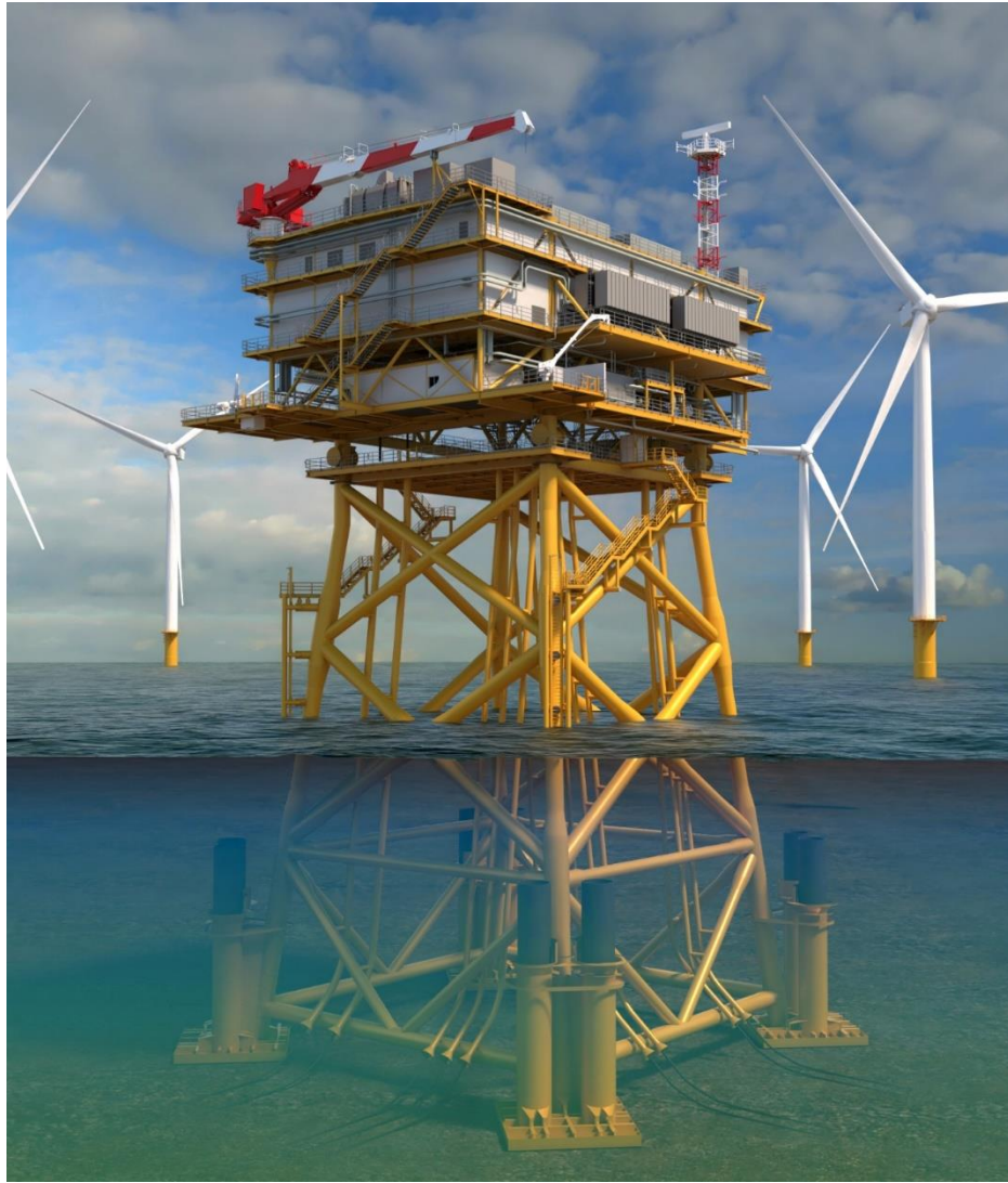
Artist's impression of the offshore substation platform solution for the Empire Wind offshore wind project (Image: Equinor, all Rights reserved)
