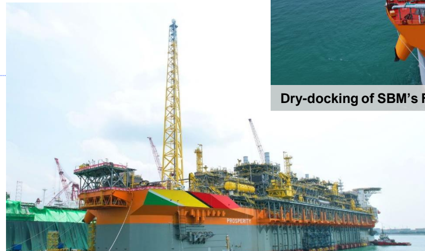
Delivery of SBM's FPSO Prosperity, the third of four FPSOs Seatrium is undertaking for deployment in Guyana
