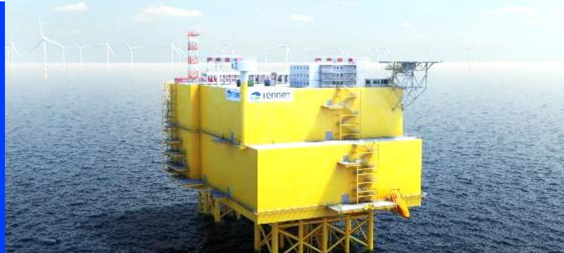
TenneT's 2GW HVDC Offshore Converter Platforms for the Netherlands
