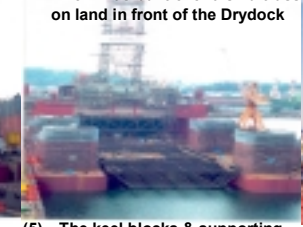
(5) The keel blocks & supporting truss in position. Skidding beam of 188 metres
