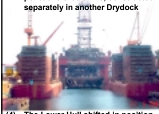
(4) The Lower Hull shifted in position in Drydock prior to skidding and mating operations
