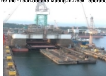
The fully assembled semi-submersible ready to float out
