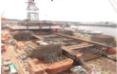
The lower pontoons towed in position in Drydock
