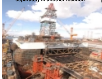
The Upper Hull fully skidded onto the lower pontoons
